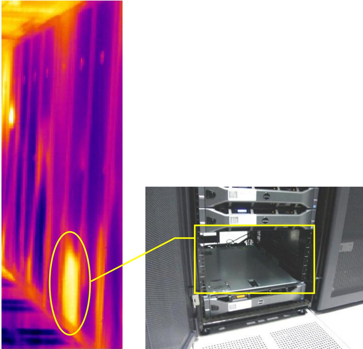
**Figure 3. Thermal Effect of Not Using a Blanking Panel**
